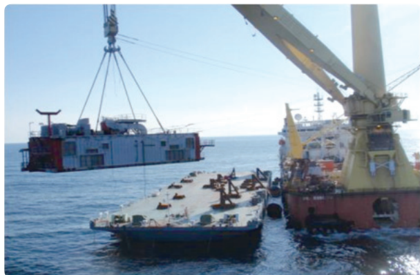
Removing above-water structures of the platform
